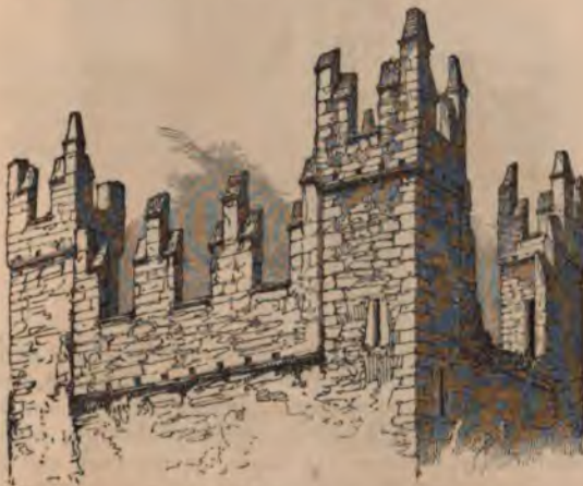
Irish Stepped Battlement and Water-drains.
